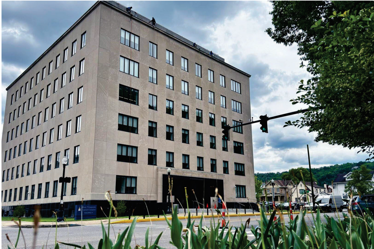
Building 4 at the West Virginia State Capitol Complex, where PDS moved in March of 2025.
